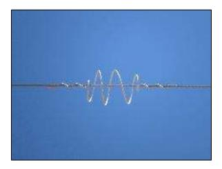
Photo 1 Bird diverter on the earth-wire
